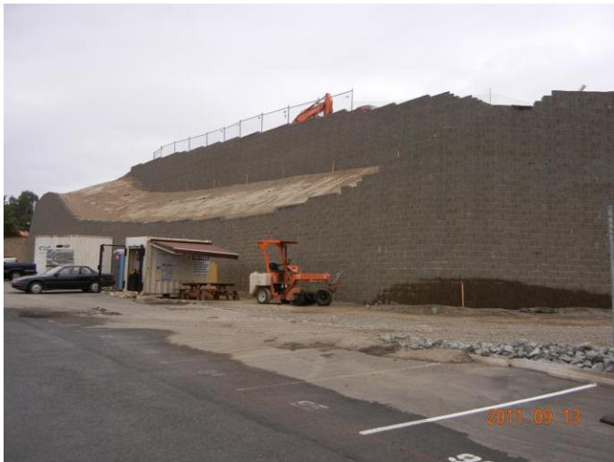
All walls have designed drainage; however, MasterPark was unique in that 15 acres of parking lot run off was purposely directed to the retaining walls. Because, contained within the balance of the wall structure were 50 - 30-foot vertical catch basins, 20 feet on center, that drained away the run-off. Additionally, there were French drains between each vertical catch basin. There is 2 to 1 sloped landscape zone wedged between 2 - 16 foot tiered walls and bookended by 2 - 30 foot corners.
