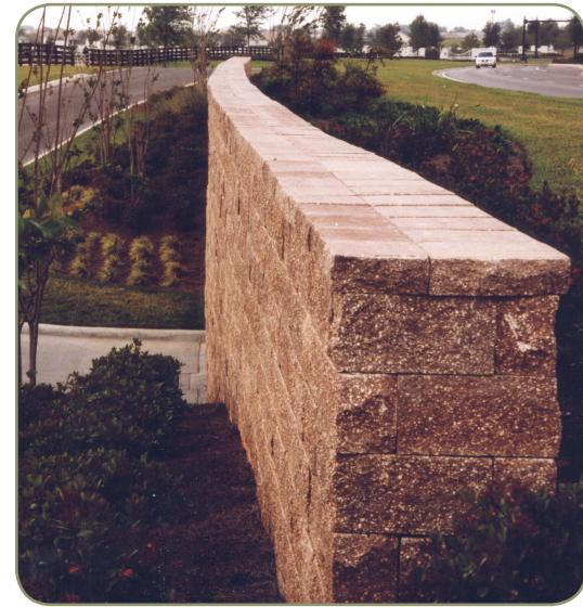
Using a combination of GravityStone Fat Face, GravityStone Thin Face and Gravity Stone Anchor Blocks, ACP installed a total of 20 tunnels with four walls each, ranging in height from 1 ft. to 14ft. To achieve the aesthetics, Falls' crew tumbled the GravityStone Thin face block until it took on a time-worn look and feel." I don't know of any other product on the market you can do that with," says Falls.
